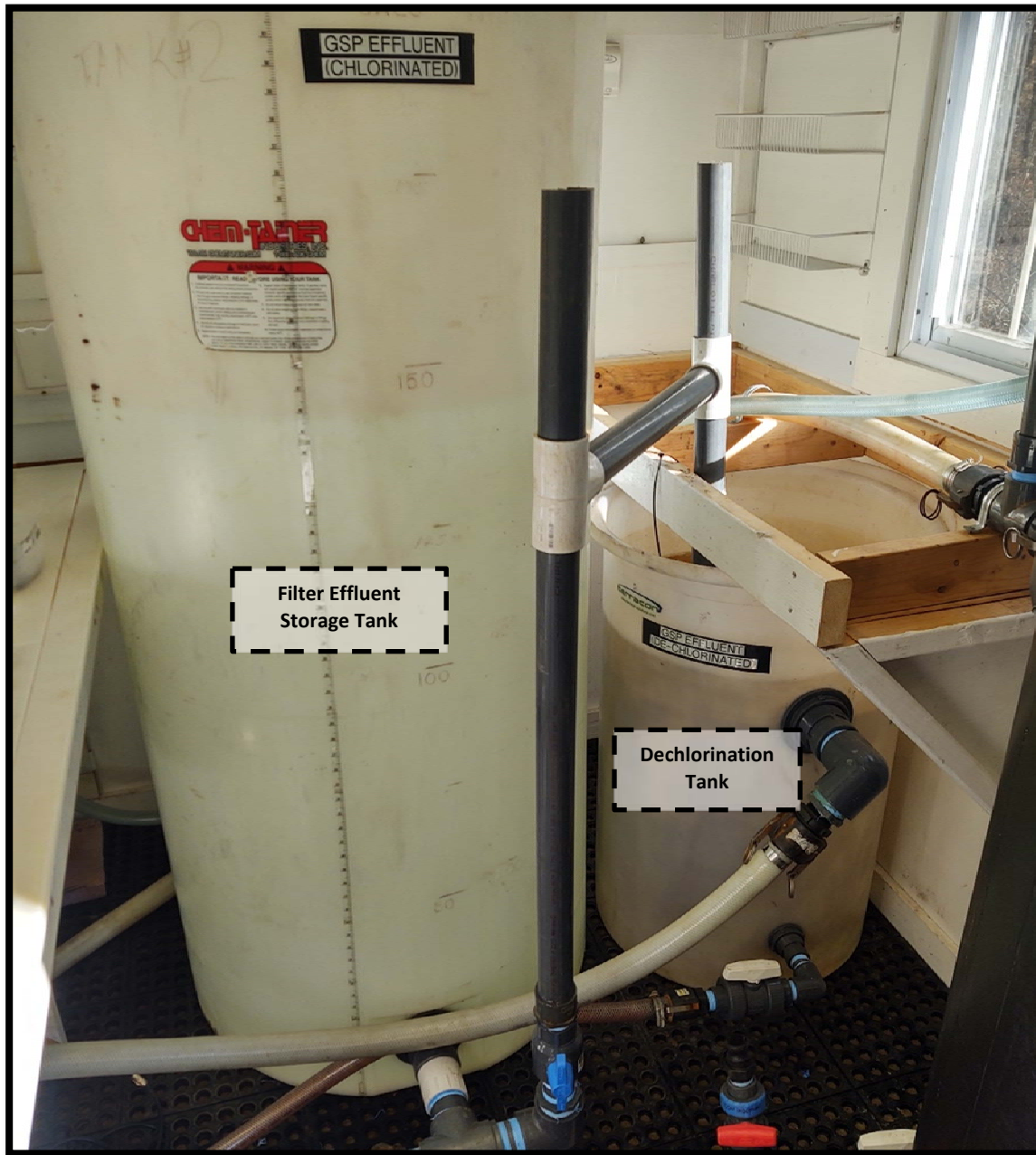
Figure 2.13: Pilot Effluent Tank and Dechlorination Feed Tank
