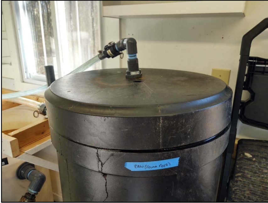
Figure 2.02: Raw Water Break Tank
