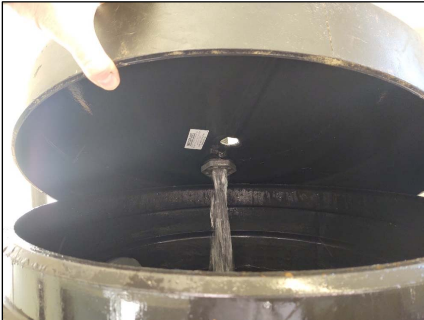
Figure 2.03: Air Gap on Raw Water Break Tank
