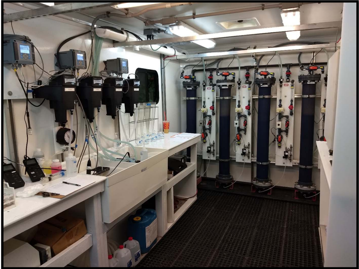
Figure 2.05: Interior of Pilot Filtration Trailer
