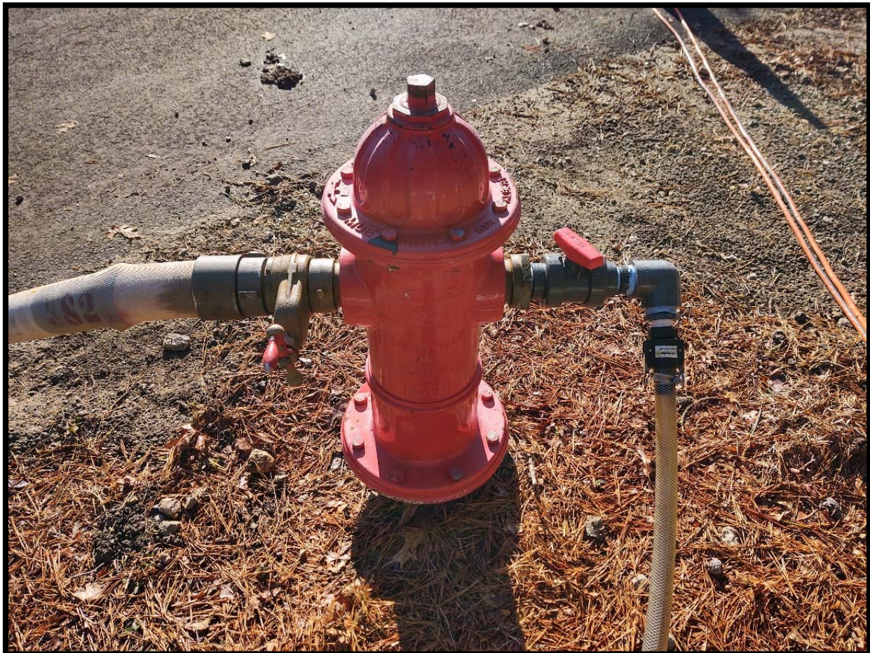
Figure 2.01: Well #5 and #2 Raw Water Connection
