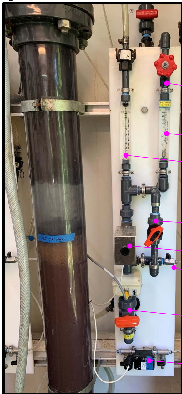
Figure 2.09: Pilot Filter with Flow Control Panel
